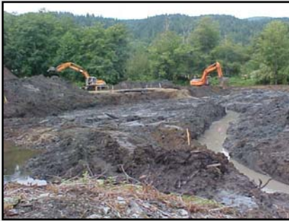
Early stages of construction
